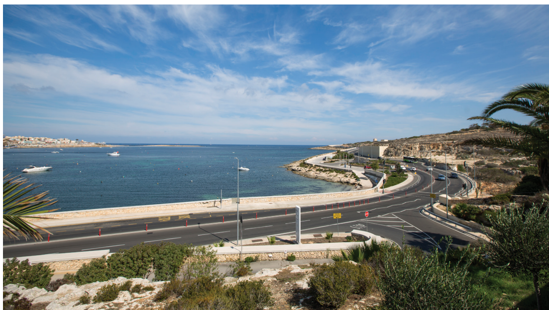
Upgrade Ten-T road Network, Malta
