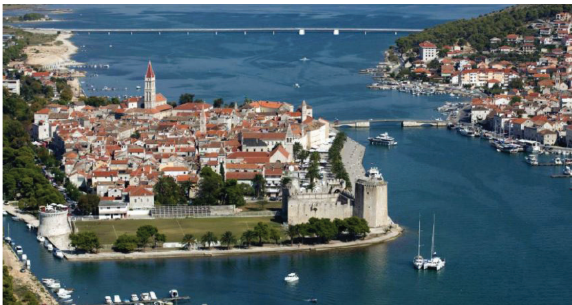
Construction of the bridge - Čiovo island in Trogir with access roads, Croatia
